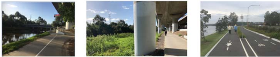
Possible “safe” separated sharing of the same Active Transport Corridor Space beside the Moonee Moonee Ponds
